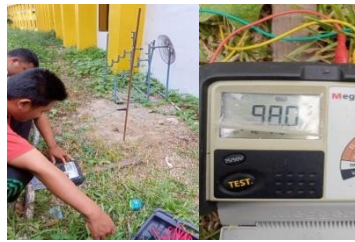
Figure 4. The measurement process using a Mega Ohm Meter (Megger)
